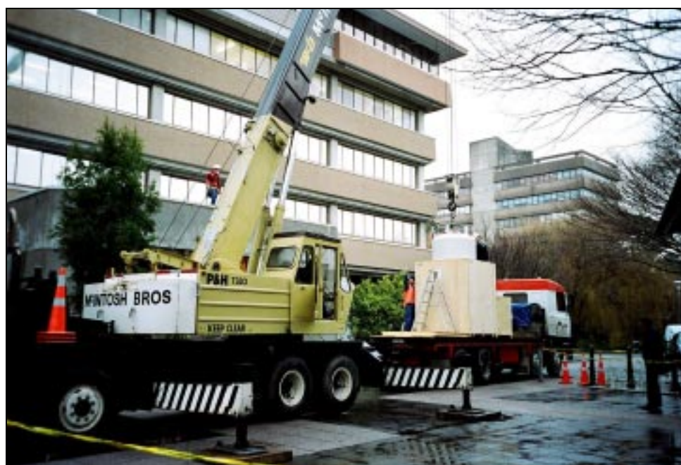
700 MHz magnet being hoisted from the packing case
