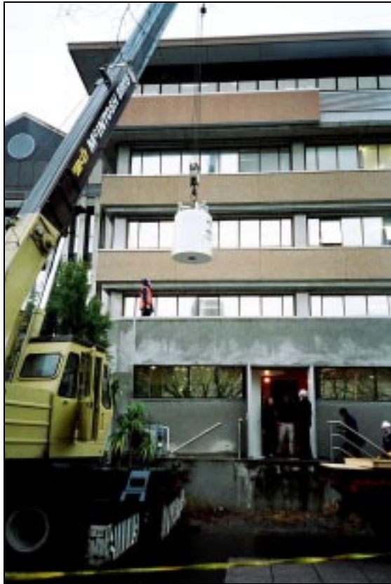
The magnet is aligned prior to lowering through the roof opening watched by the Minister for Research, Science and Technology Hon Pete Hodgson
