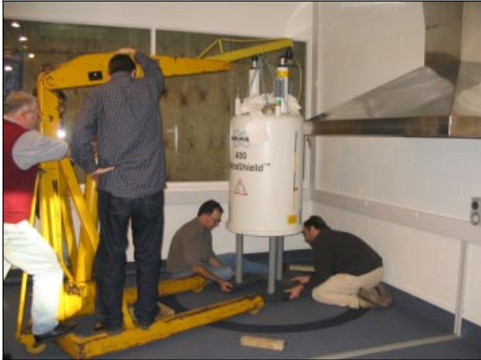
Bob Parsons and Rob Ward keeping an eye on the progress
